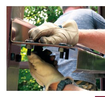
Engineered cees and zees **bolt together** with solid steel plates to give Sierra<sup>™</sup> Series its strength.
